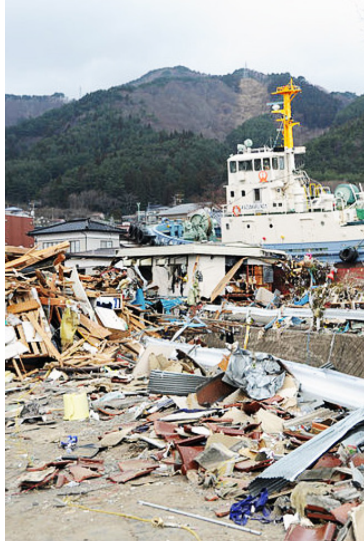
Earthquake damage in Japan.
